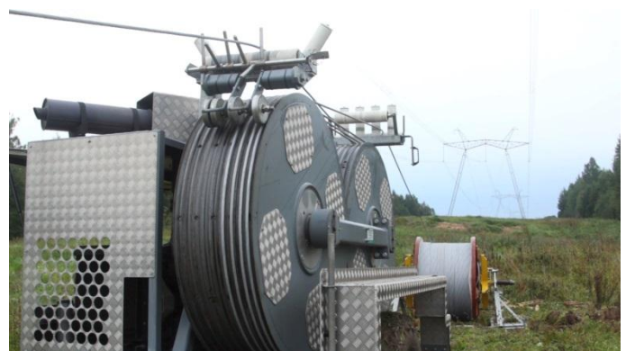
Building fiber-optic communication lines (FOCL)
