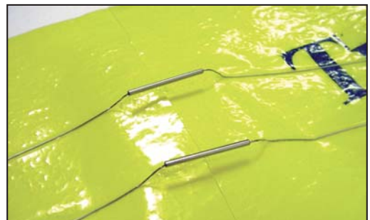
Connection of the tape using the crimps. If the tape wires are not installed correctly then the signal may not pass from join to join.
